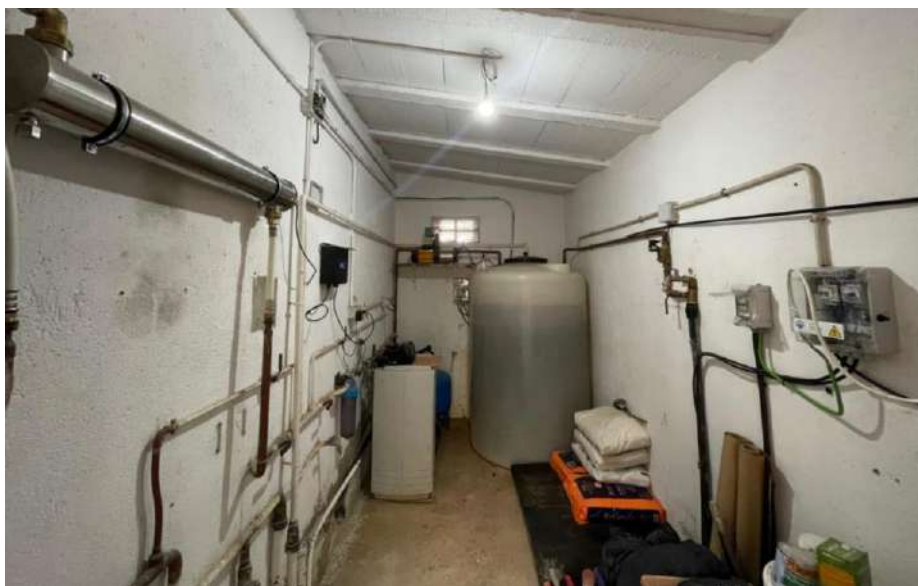
INTERIOR COS ANNEX
